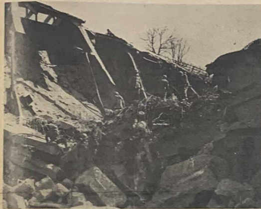
A group of 111th Engineers examine the wreckage of the bridge preparatory to constructing a bypass on the road leading north from Kaiserslautern.
