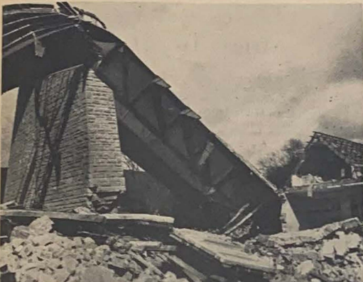
German engineers demolished this overpass along the autobahn running to Kaiserslautern from the west.
